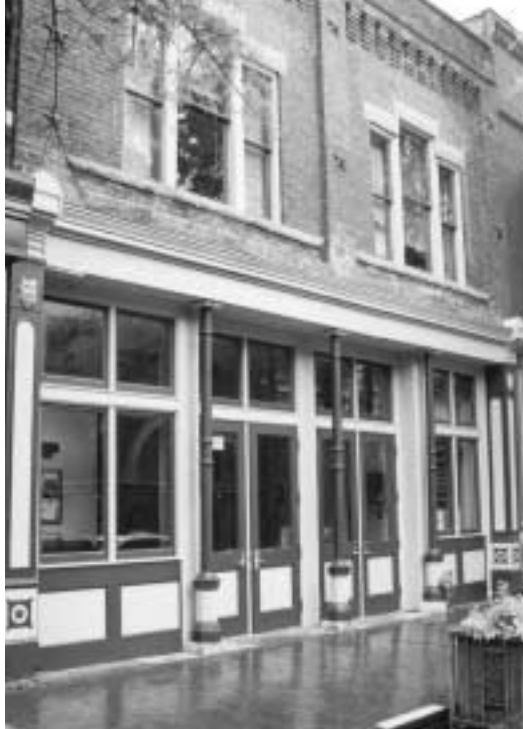
THE MARKET HOUSE THEATRE COMPLEX IN PADUCAH, KENTUCKY AFTER RESTORATION WITH TRANSPORTATION ENHANCEMENT FUNDS. PHOTO: RAY BLACK & SON, INC.
